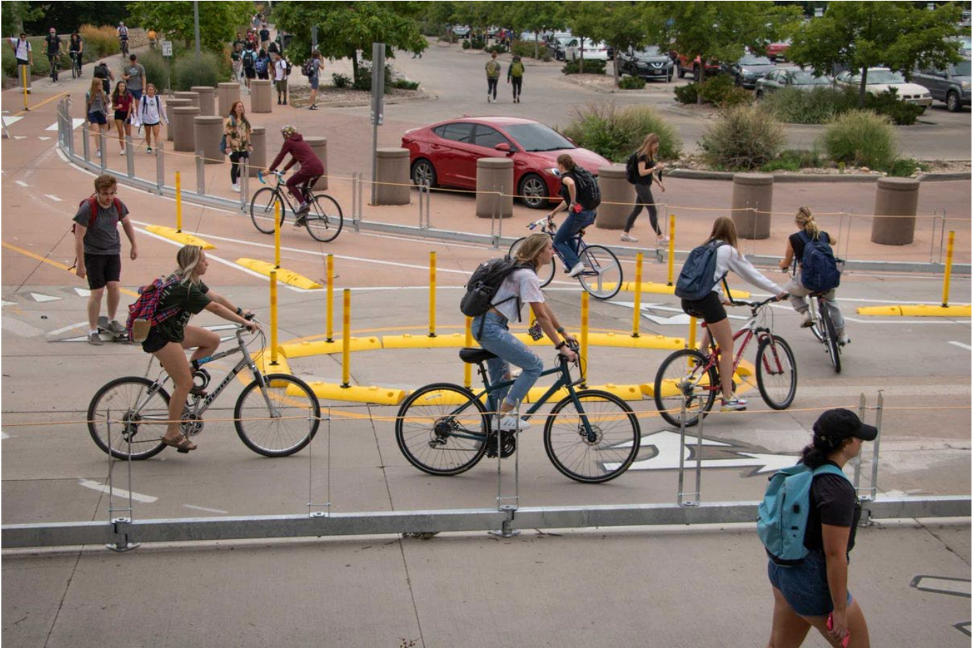
A bicycle roundabout created at CSU with rubber curbing and flexible bollards is an example of an innovative treatment using low-cost materials that are easily adjusted. Source: CSU.
